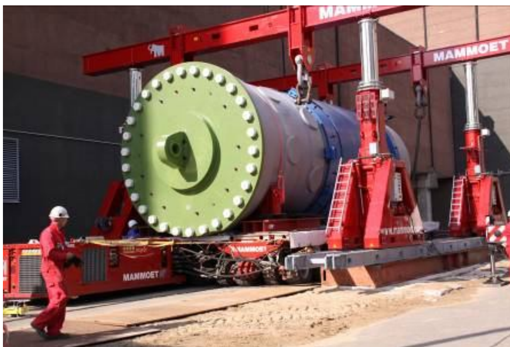
Fig. 1.6.1.1.3-1 Transportation of the RPV
